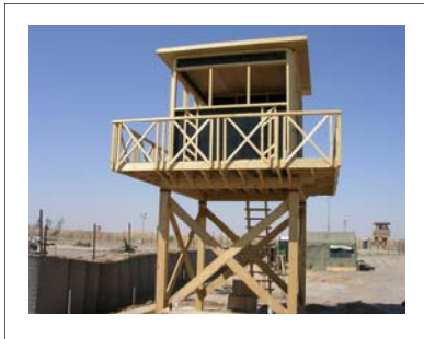
A new tower out at the TIPF
